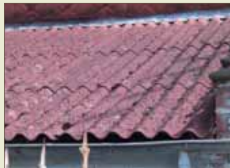
Dakgolfplaten in asbestcement
