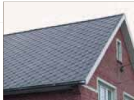
Dakleien in asbestcement
